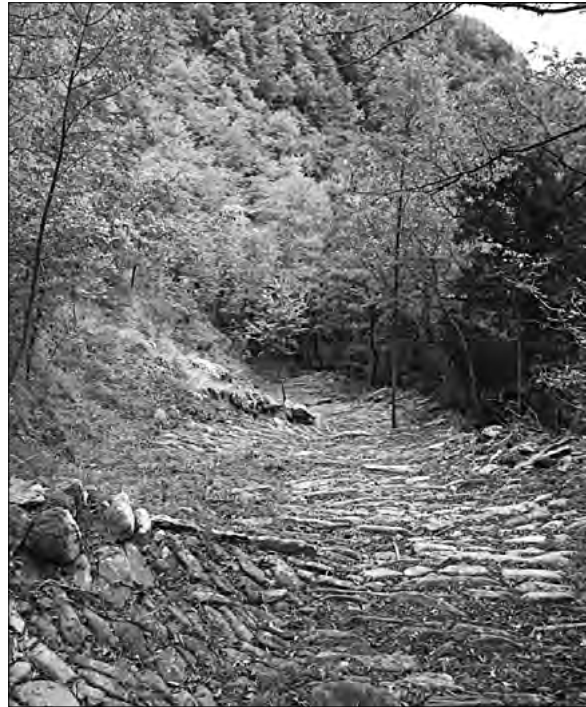
Fig. 4. The «Scaleri». A medieval mule track with transverse drainage channels near a derelict xenodochium , Cirone pass, on the Francigena network between Pontremoli and Monte Bardone.
